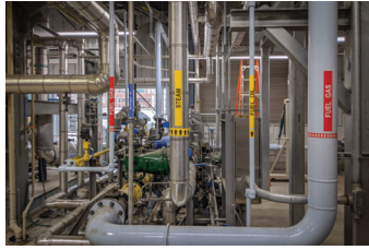
Inside the Denver Steam Plant, natural gas is burned to boil water to serve about 120 downtown buildings with steam.
