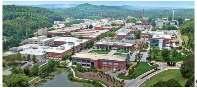
Aerial view of Oak Ridge National Laboratory.
