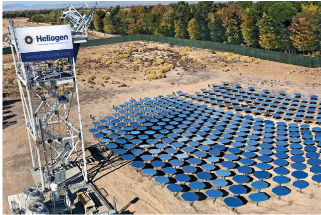
Heliogen's demonstration tower in Lancaster, Calif.
